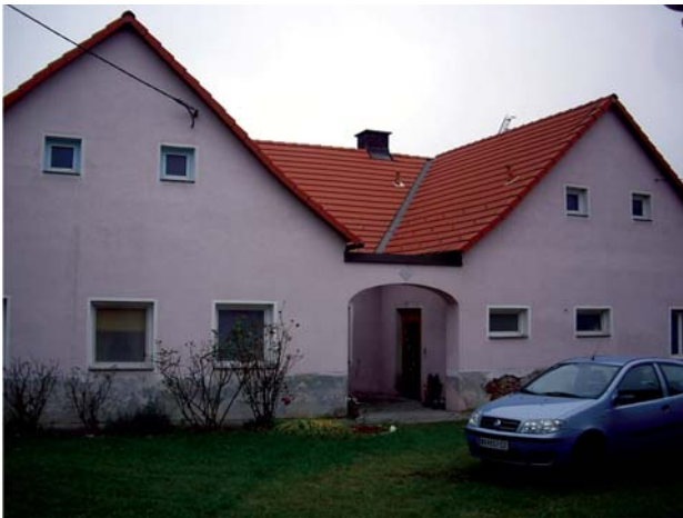
Figure 6: Rear view of House No. 48, in 2008 (photograph by the author).
